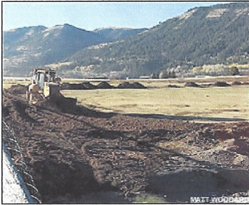
An irrigation channel — similar to ones that drained Garden Creek — is filled in with soil.
